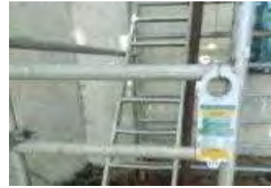
System of Inspection and tagging of Scaffolds for safe Use.
