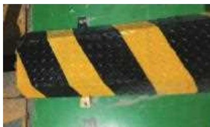
All area with pipelines above floor covered with flat surface and hazard marking done.
