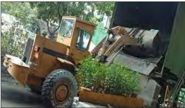
← Earth moving equipment used for material shifting at Plant
