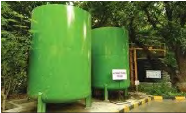
← Metal Tanks for Admixture storage
