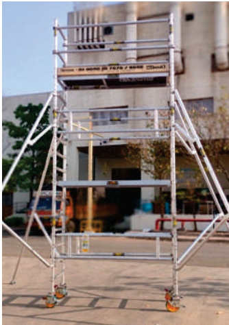
CEHS Approved Standard Scaffolding with Safety Tags with Trained and certified Scaffolding erector (30) and Inspector (4)
