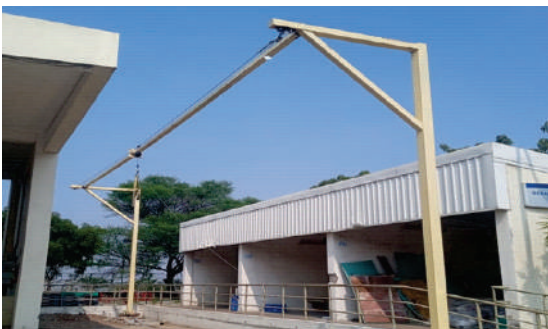
Implemented lifeline system in Scrap Yard, WMS Scrap, LG Dock, and OCM Dock.
