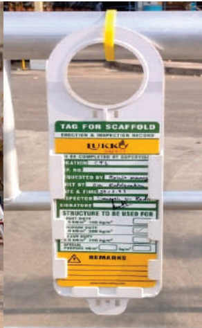
CEHS Approved Standard Scaffolding with Safety Tags with Trained and certified Scaffolding erector (30) and Inspector (4)
